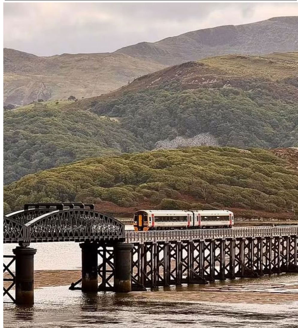
Barmouth Bridge Cambrian Coast Railway Line
