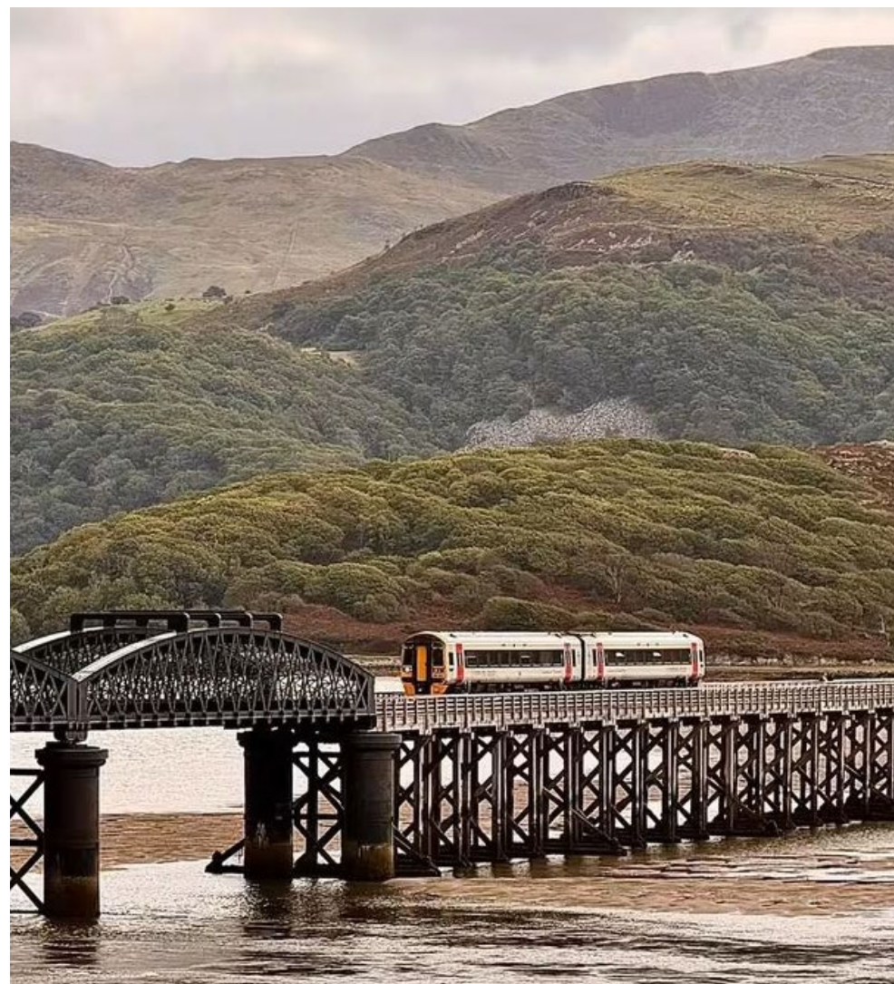
Barmouth Bridge Cambrian Coast Railway Line
